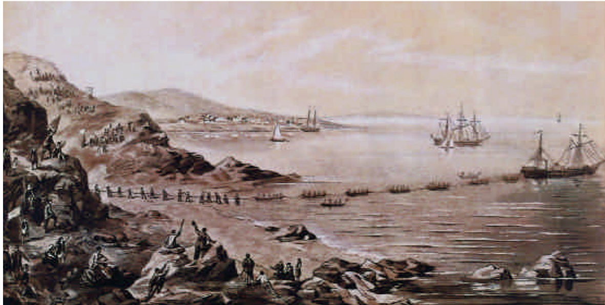
The first attempt to lay a transatlantic submarine telegraph cable. Valencia island (Ireland), 1857. (Contemporary engraving).
