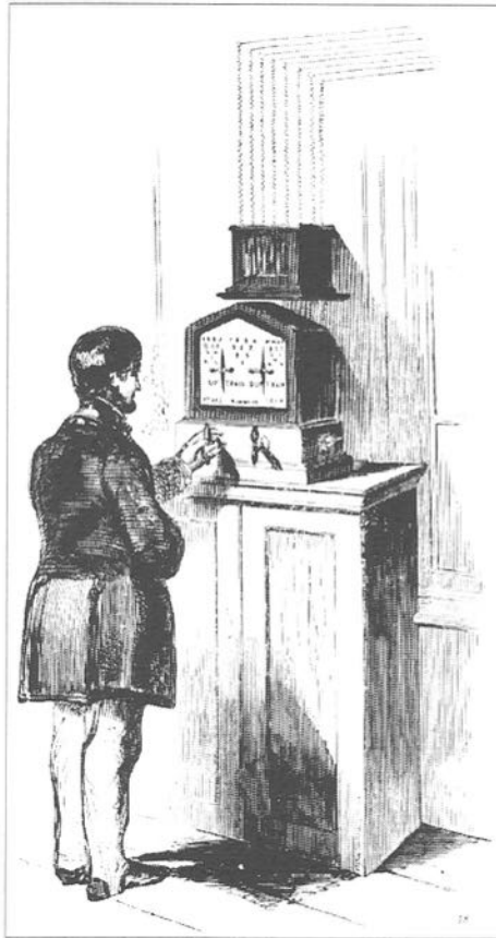
Figure 5. The cabinet shows two single needle instruments, one for the 'up' and the other for the 'down' line of the railway. For this only two wires and an earth connection will have been needed. For a five needle Wheatstone instrument four wires and an earth were required. However eight wires are shown suggesting that originally there were two Wheatstone five needle instruments (Pictorial Times 1845).
