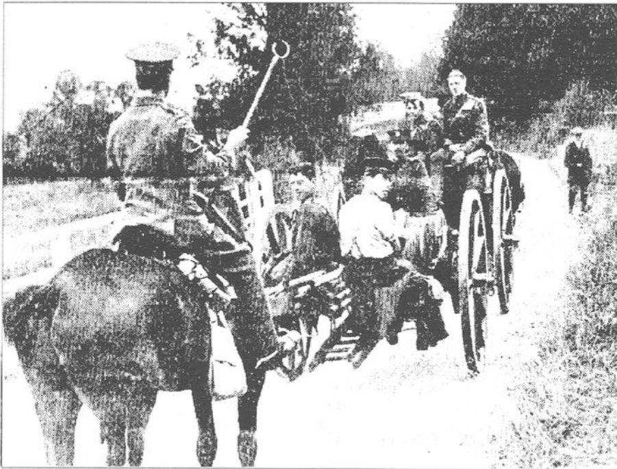
Figure 9. An outrider guides the wire with a crook stick so that it is laid to the side of the road.
