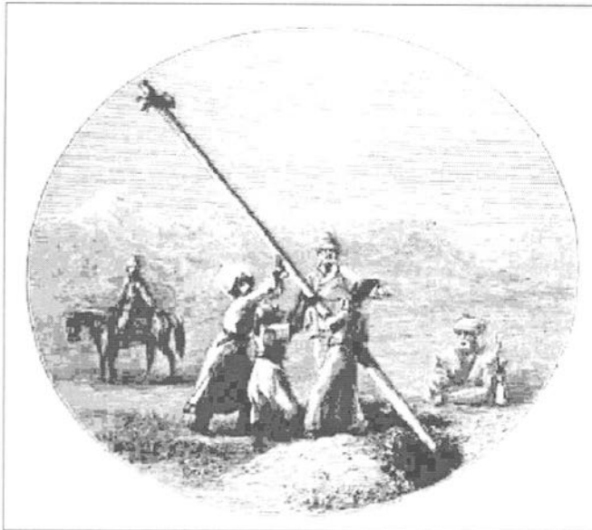
Figure 11. Erection of a telegraph pole in the East. Goldsmid 1874.
