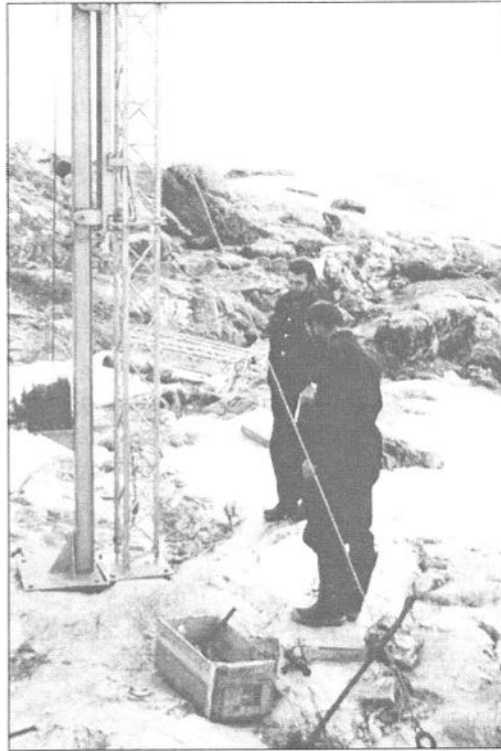
John McKenzie and Graham Currie repairing radio masts, Wilkes 1963.
