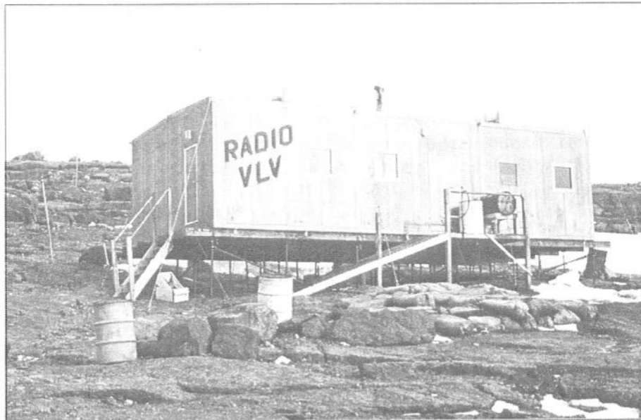
Radio VLV, Mawson radio hut, constructed 1963.
