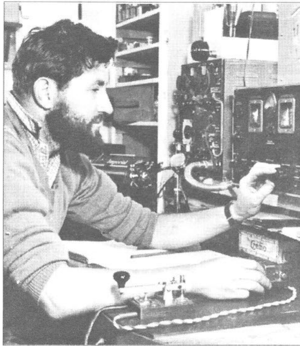
Mawson 1954. Bill Storer using amateur equipment. Left is AT5 transmitter, right is Hammerlund receiver.
