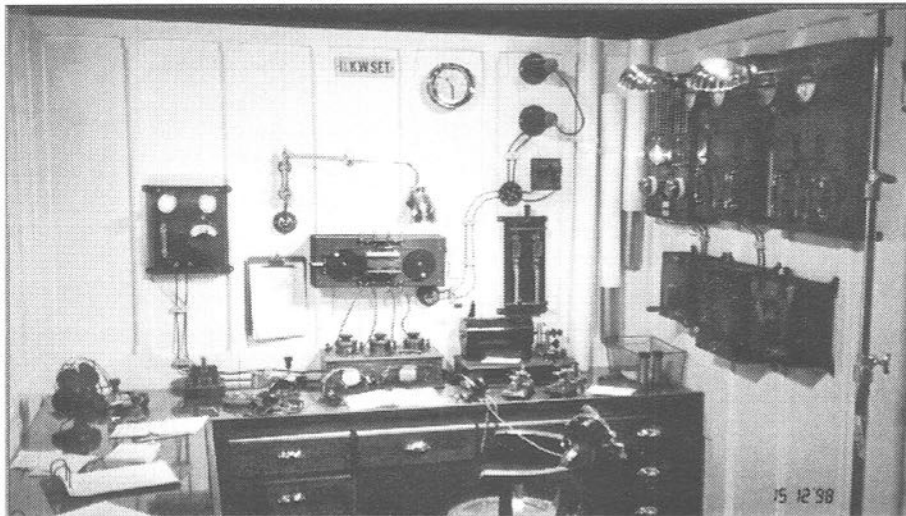
Fig. 2: Re-creation of the Titanic's wireless room
