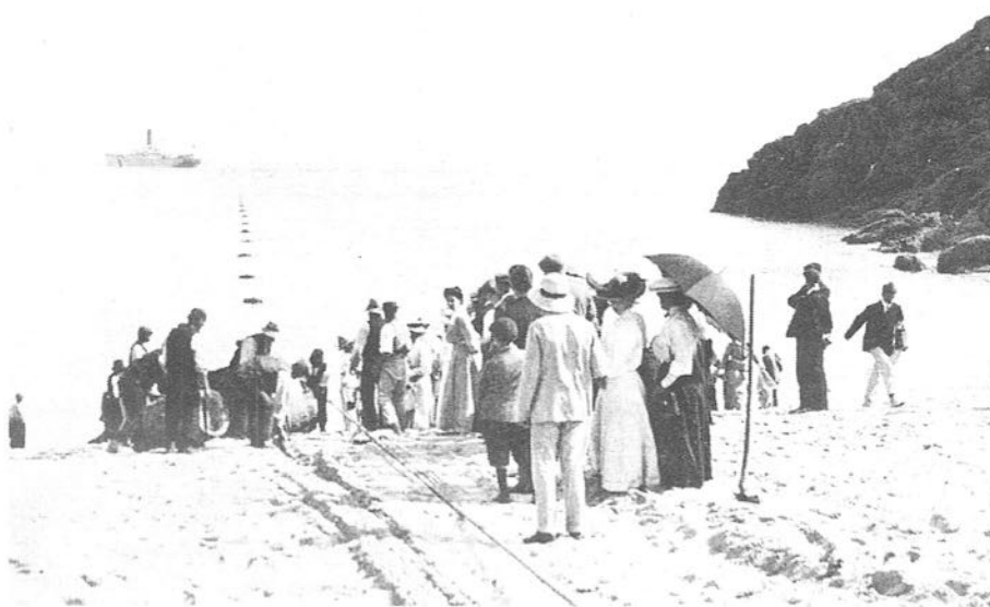
Bringing a cable ashore at Porthcurno, from the Azores, 1906
